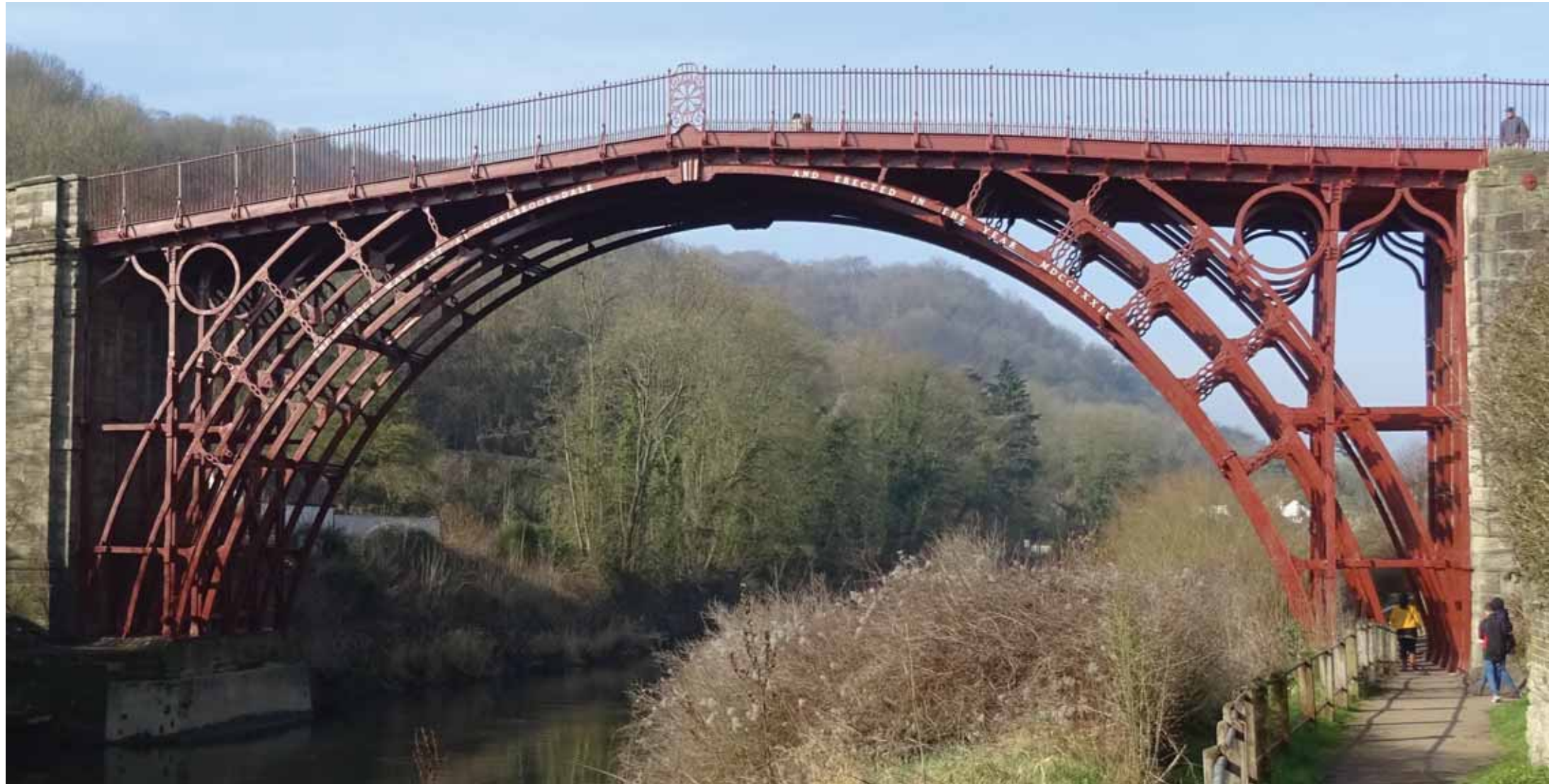
The Iron Bridge 1781 Thomas Farnolls Pritchard and Abraham Darby III
